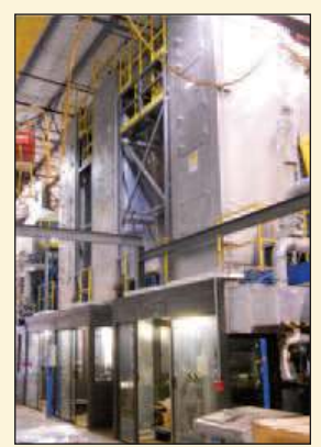
Coating Stations on Bottom, Gas Fired Ovens on Top
