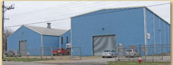
Building located in Blytheville, AR
